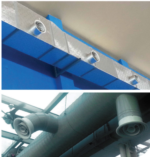
Exposed duct system Installation c/w RRD
